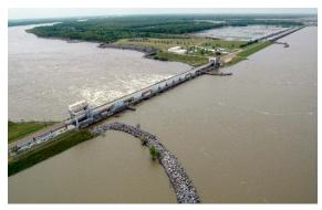
the Mississippi and Red rivers. The Old River navigation lock was constructed to allow navigation between the Mississippi, Red, and Atchafalaya Rivers. A dam was constructed north of the lock across the natural stream Old River, preventing the Mississippi River from changing its course.
