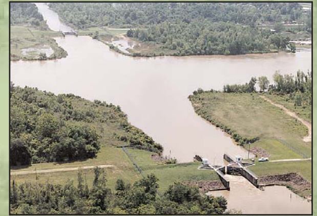
East and West Calumet Floodgates
