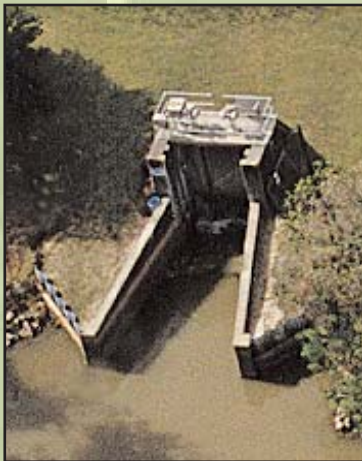
Bayou Darbonne Control Structure
