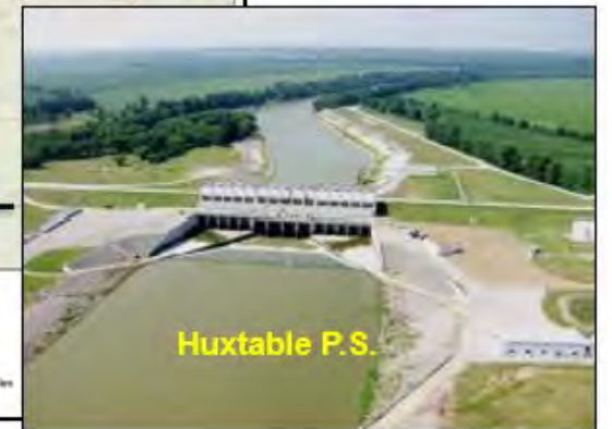
Ditch 81 Control Structure
